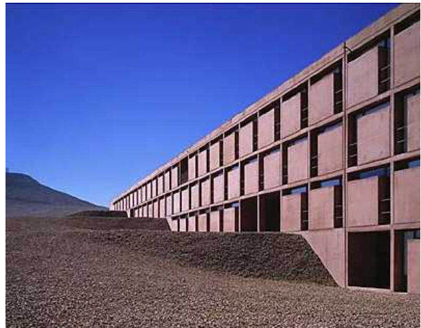
Chile: Hotel and Information Centre for the European Southern Observatory at Cerro Paranal Site-mixed concrete, pigmented with Bayferrox® 600 N
