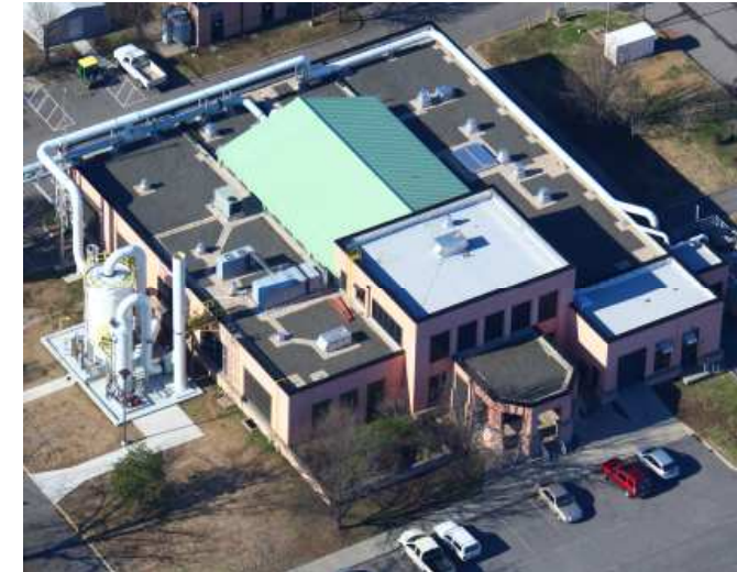
Hampton Roads Sanitation District - VIP Plant, Norfolk, VA
