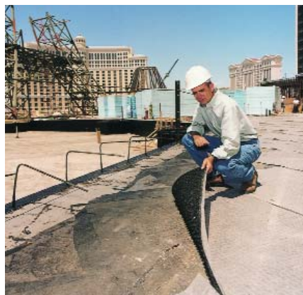
Enkadrain offers excellent drainage for planters and plaza decks. By replacing gravel, it reduces weight and increases soil area for a healthier root mass.
