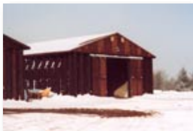
Salt Storage Buildings
