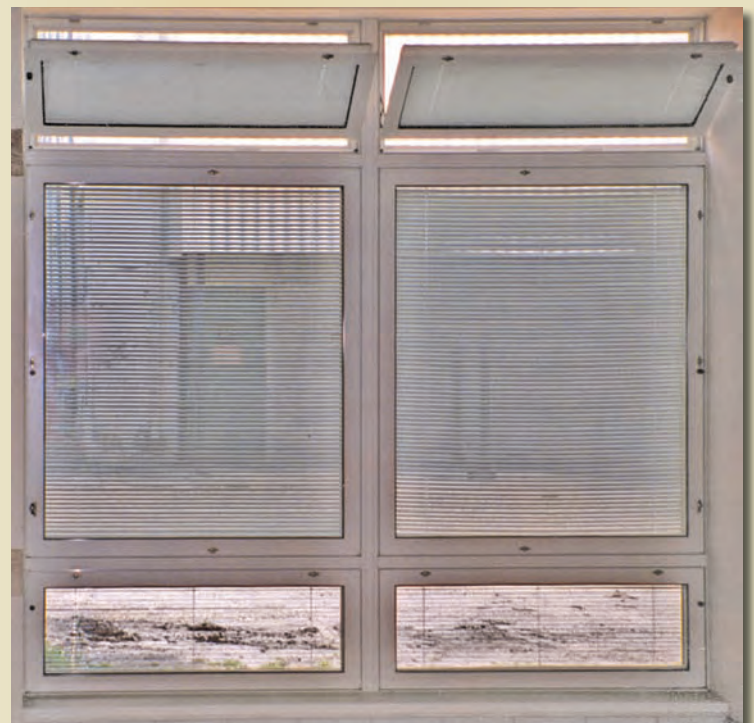
Acute Care Facility - Portsmouth, VA
