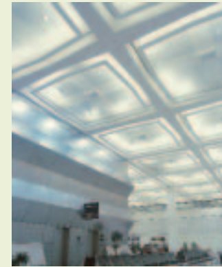
Project: Bush Intercontinental Airport Location: Houston, TX Architect: Gensler, Houston Product: Hook-On
