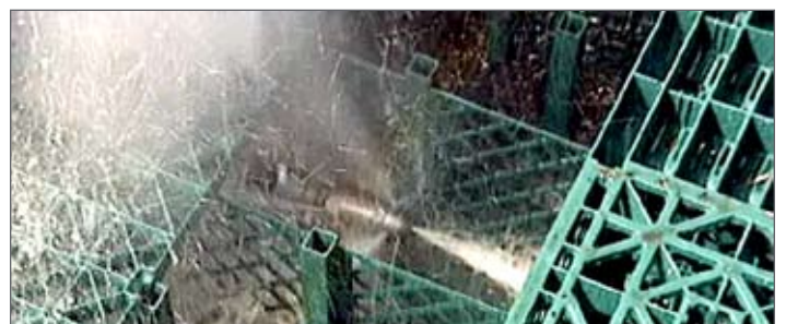
Figure 10: The pressure washing nozzle is moved along the entire length of the Stormbloc™ row
