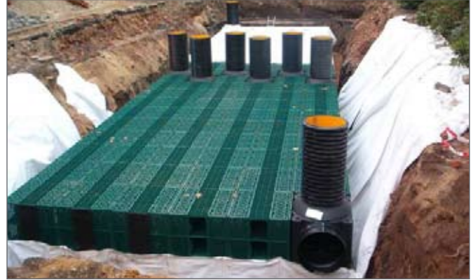
Figure 5: One Stormbloc™ Inspect is used per row of Stormbloc™ blocks
