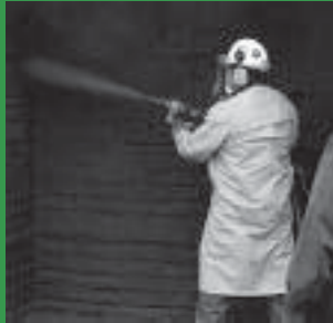
Cementitious Structural Repair
