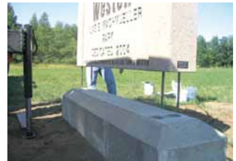
Allow our crane to set the sign onto the footings.
