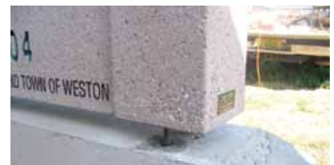
Following placement, secure the sign, allowing the mortar to harden.
