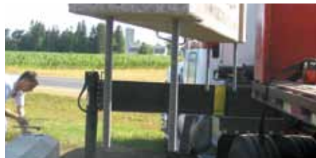
Threaded rods provide the connection with the construction and the footings constructed prior to delivery – ask about our available sign bases.
