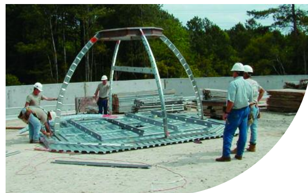
DOMES KIT BEING ASSEMBLED ON PROJECT SITE
