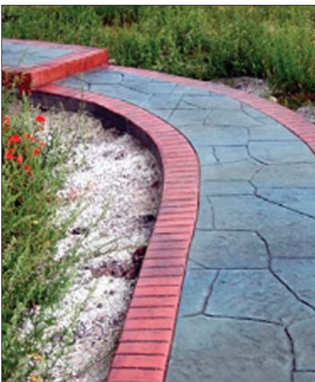
Stamped Walkway Colored with Direct Colors Pigment (Photo Courtesy of Mike Douglass)
