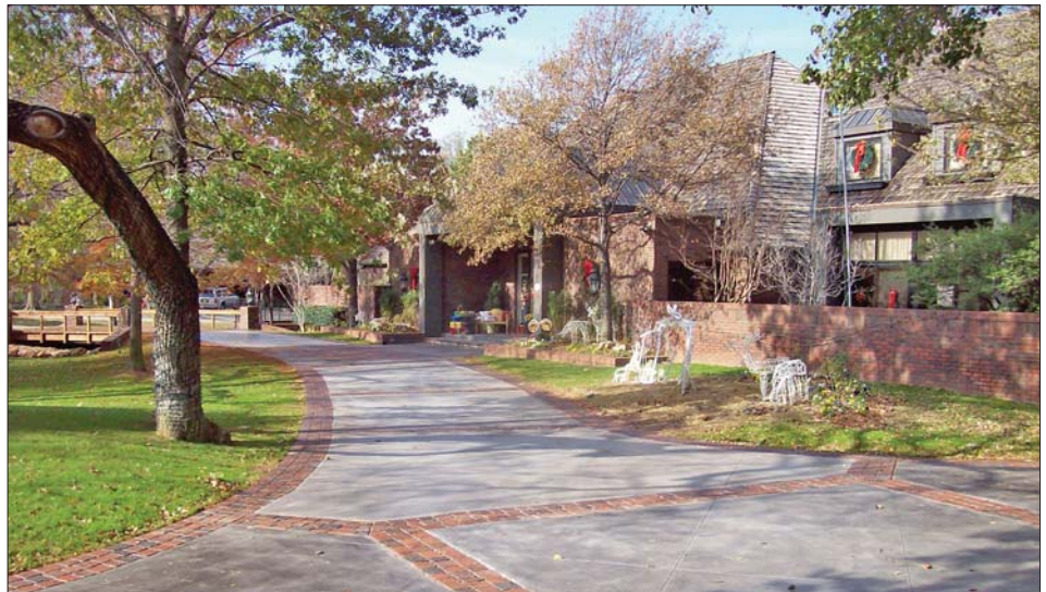
Stamped Concrete Colored with Direct Colors Inc. Pigment Dispersed in Antique Release and Tinted Sealer (Photo Courtesy of Decocrete)
