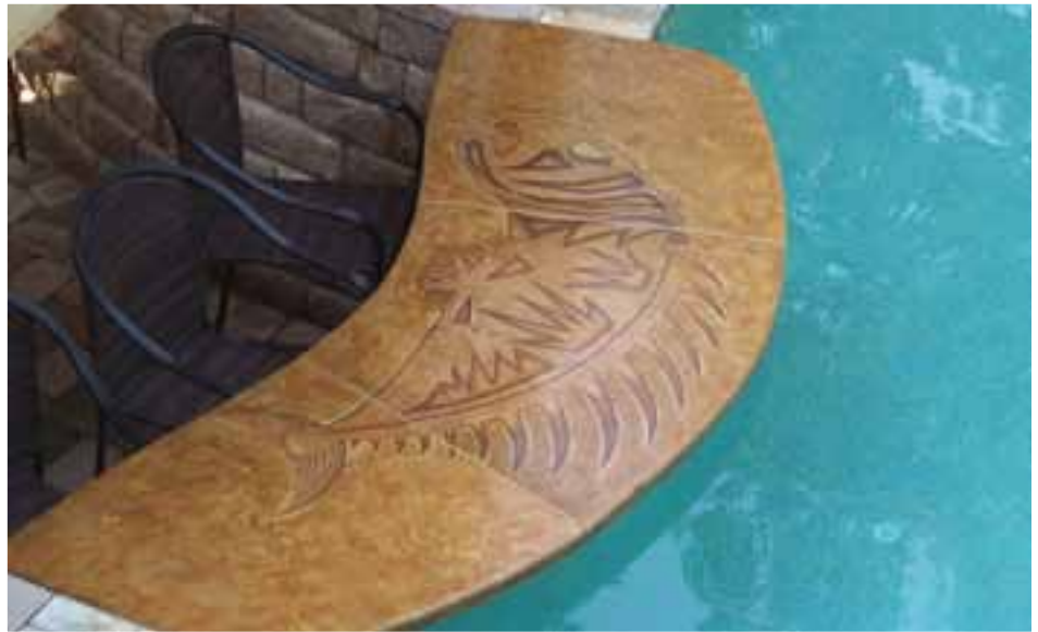
Swim-up pool bar countertop colored with 1311 Concrete Pigment, English Red Acid Stain and English Red Deco Gel (Photo Courtesy of Susan Turfle)
