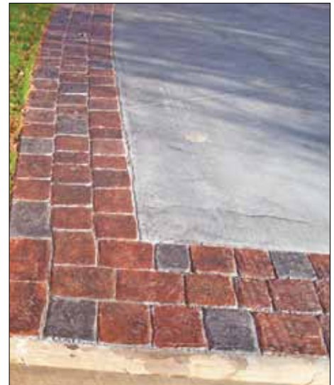
Close-up of stamped concrete walkway as shown above (Photo Courtesy of Decocrete)
