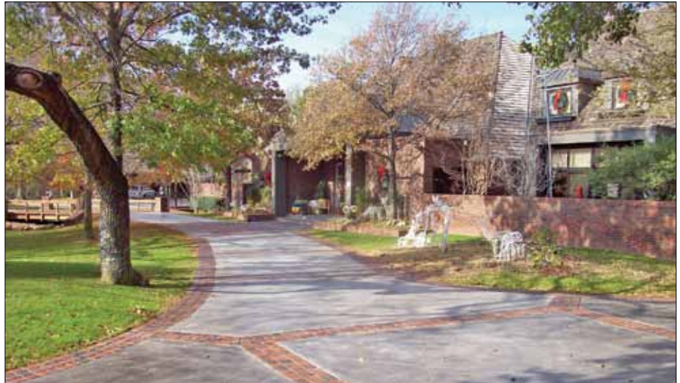
Stamped concrete colored with Direct Colors Concrete Pigment dispersed in Antique Release and Tinted Sealer (Photo Courtesy of Decocrete)
