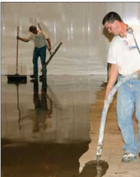
WearTop pouring over damaged concrete
