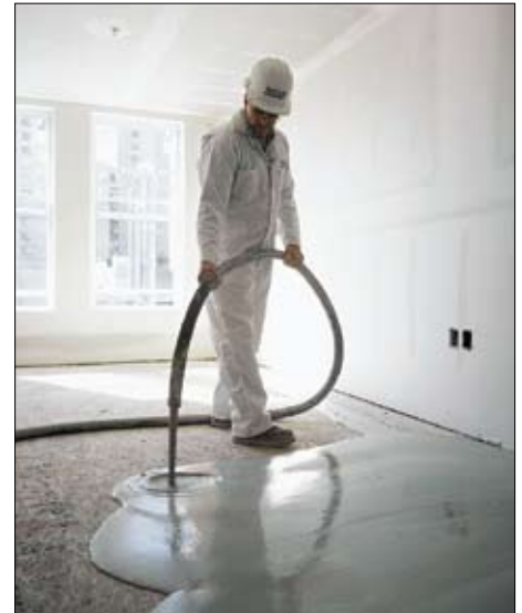
Maxxon Underlayments provide solutions for floor leveling, sound control, floor warming and enhanced fire control.
