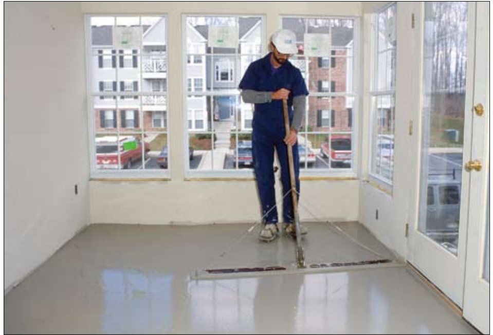
Rapid Floor® Underlayments fill cracks in the subfloor and seal perimeter joints, significantly reducing sound leaks.
