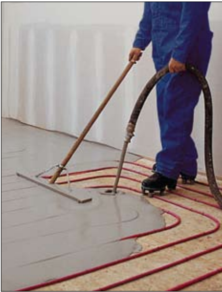
Rapid Radiant® is an ideal thermal mass for installation over radiant heat tubing or electric cables.
