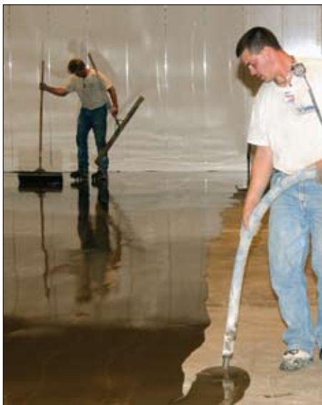
WearTop pouring over damaged concrete
