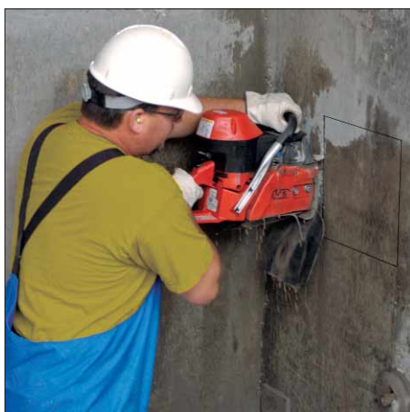
Plunge saw directly into wall.
