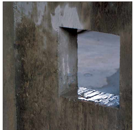
Finished 2' x 2' (0.61 x 0.61 m) opening in under 20 minutes
