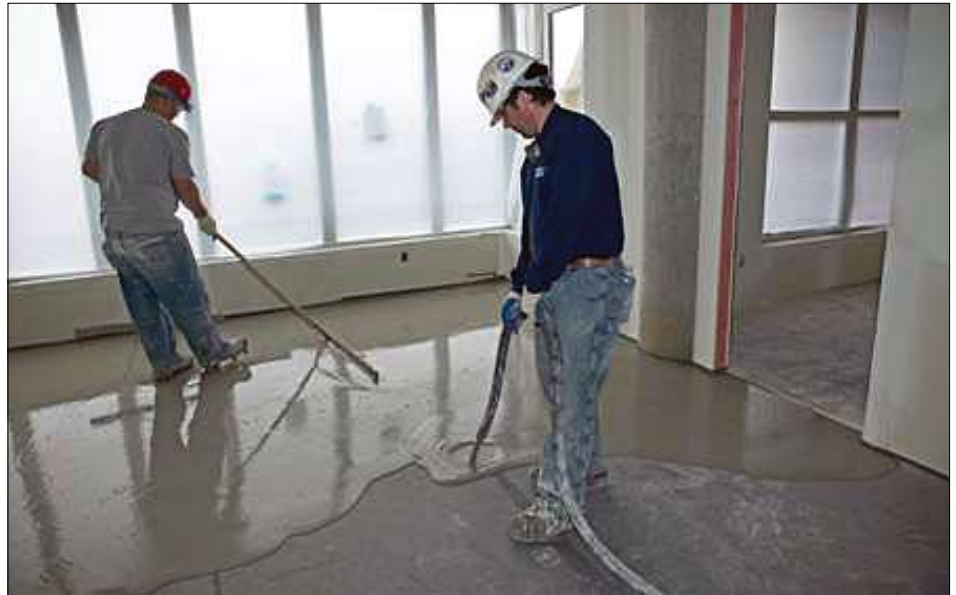
Maxxon Underlayment poured over Acousti-Mat® LP
