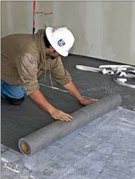
Acousti-Mat® LP attached to concrete subfloor
