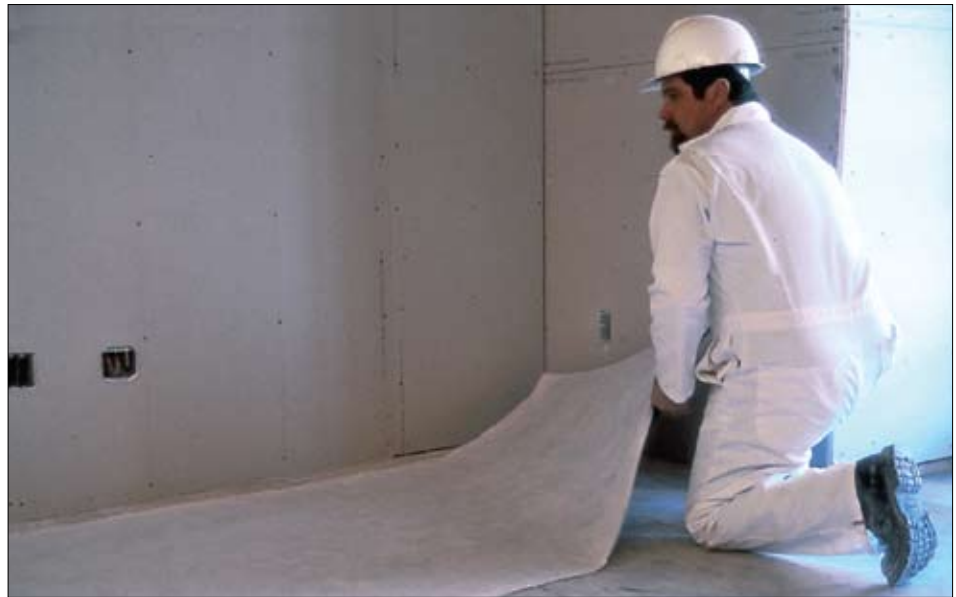
Sound mat is loose laid over the entire concrete or wood subfloor.
