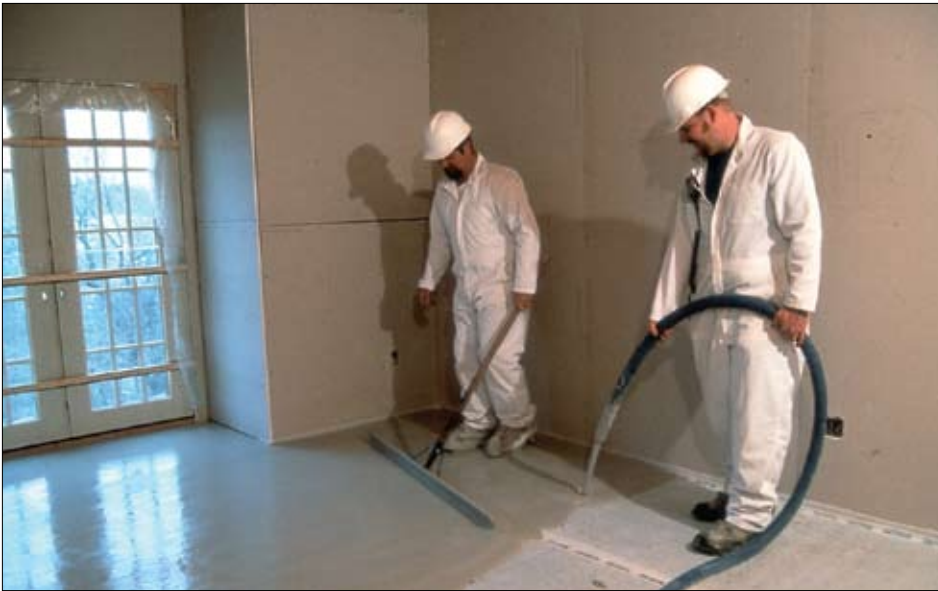
Sound mat is topped with approved Maxxon underlayment.
