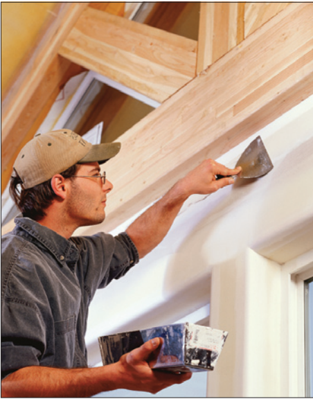
NO-COAT L Trim Install
