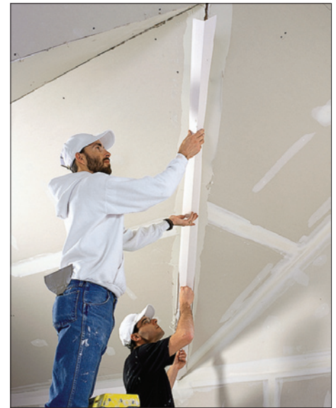
NO-COAT ULTRAFLEX Application
