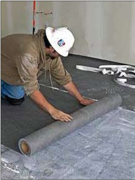
Acousti-Mat® LP attached to concrete subfloor
