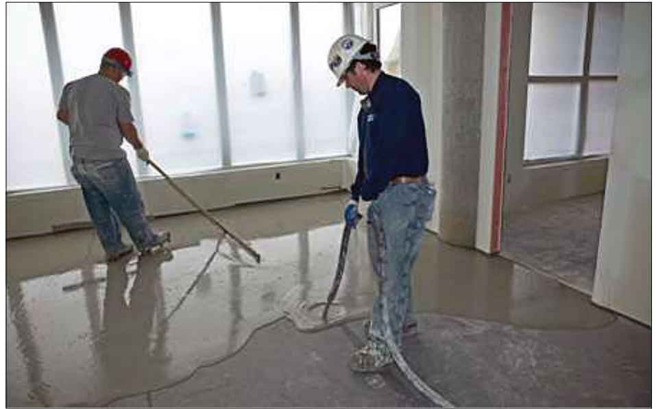
Maxxon Underlayment poured over Acousti-Mat® LP
