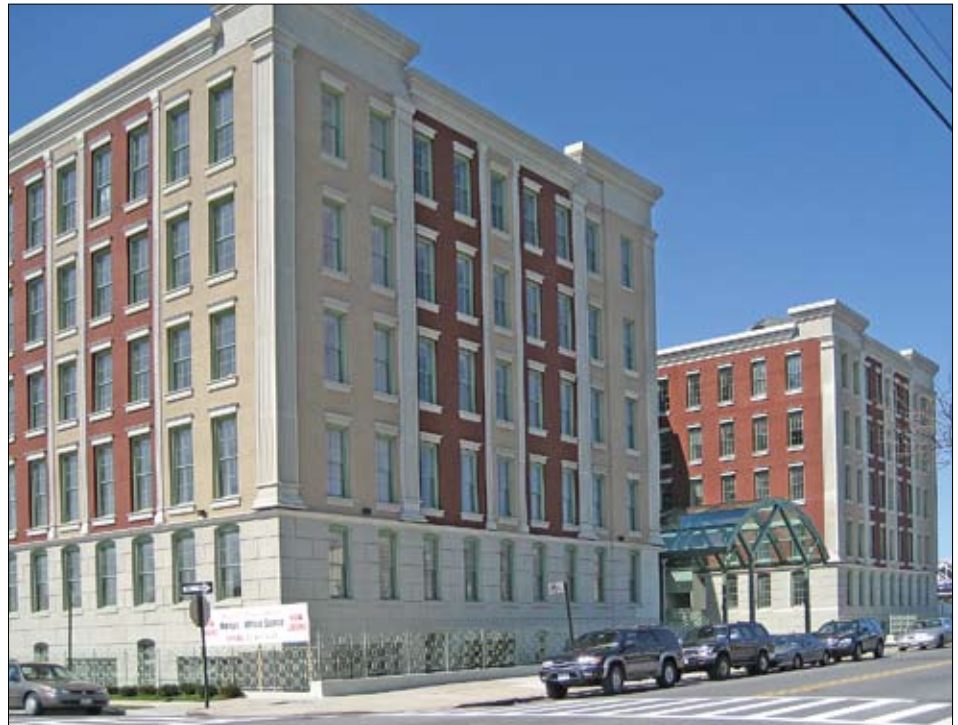
Steinway Piano Condominium Building, Astoria, New York
