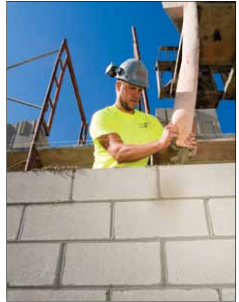
SPEC MIX SCG reduces labor by eliminating consolidation and reconsolidation of masonry grout.
